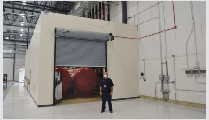
Foam equipment room shown here was constructed to house main and reserve foam tanks, system risers, fire pumps and controls.
