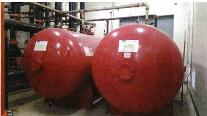
Two 2,600-gallon bladder tanks containing a total of 5,200 gallons of RE-HEALING 3% Fluorine-free foam.
