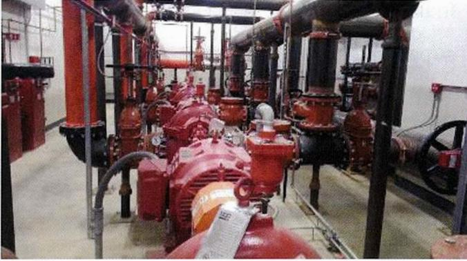
Four 2,500 gpm electric fire pumps were installed and supplied by a new 16" ductile feed into the building.
