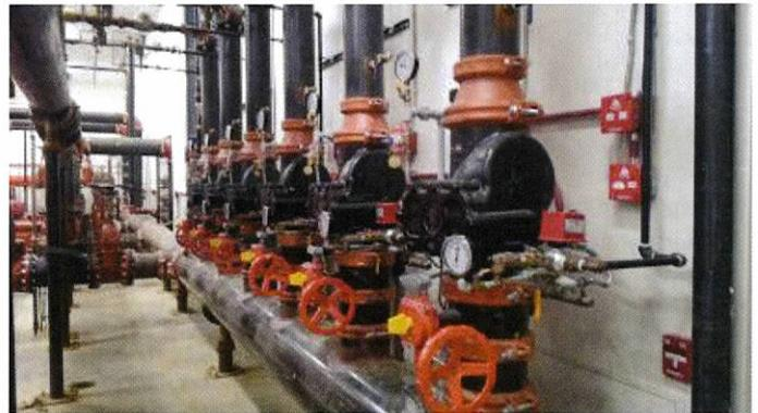
Foam-water deluge systems protecting the entire hangar floor space. Each deluge system protected an area over 9,000 square feet each.
